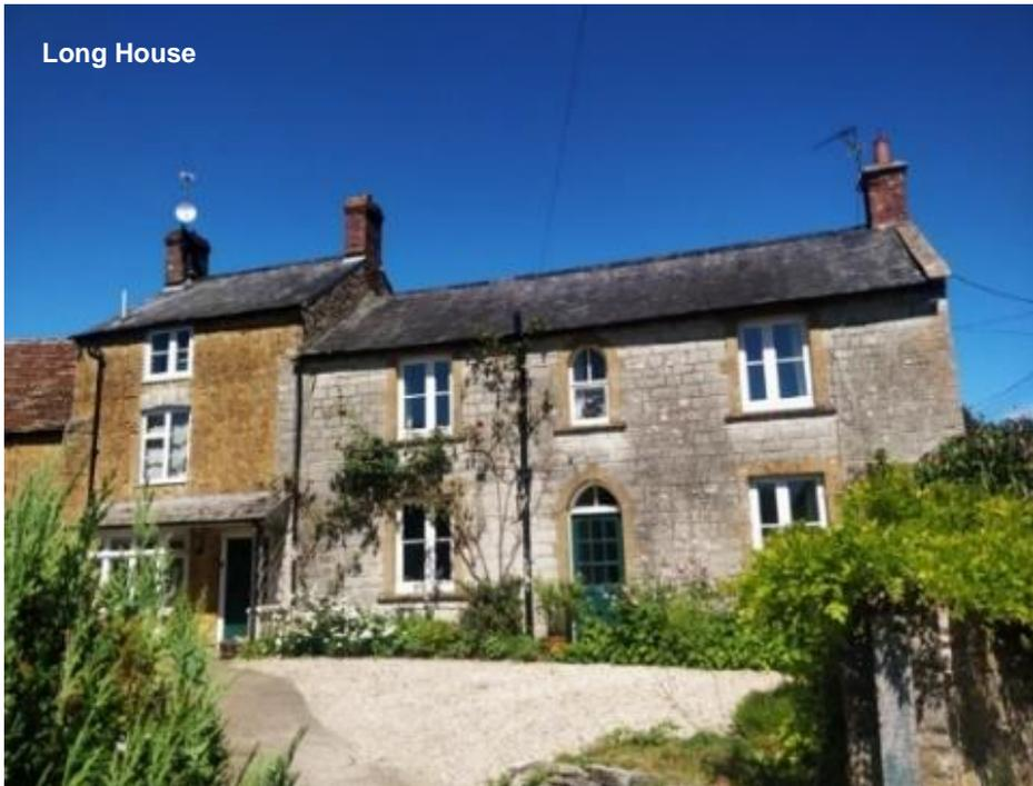
12.9 Local marl is found in fields north of Galhampton and the soil is generally a fine sandy loam. The local stone quarry at Hadspen supplies coursed, random rubble walling stone, local Lias, Cary stone and Bath stone. As a result, many of the older buildings are built from local stone or rubble, with coursed and dressed ashlar. Whilst the vast majority of houses would have been roofed in combed wheat reed thatch, Agecroft
