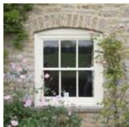
Sash window with stone arch
