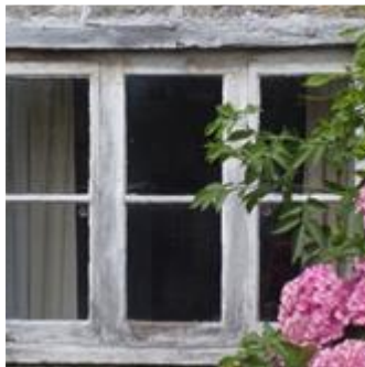
Painted casement window
