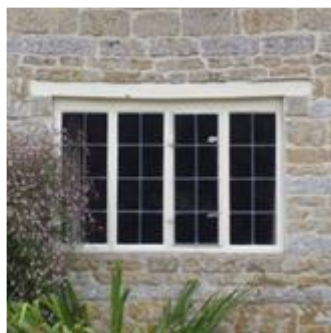
Leaded light window and polychromatic stonework
